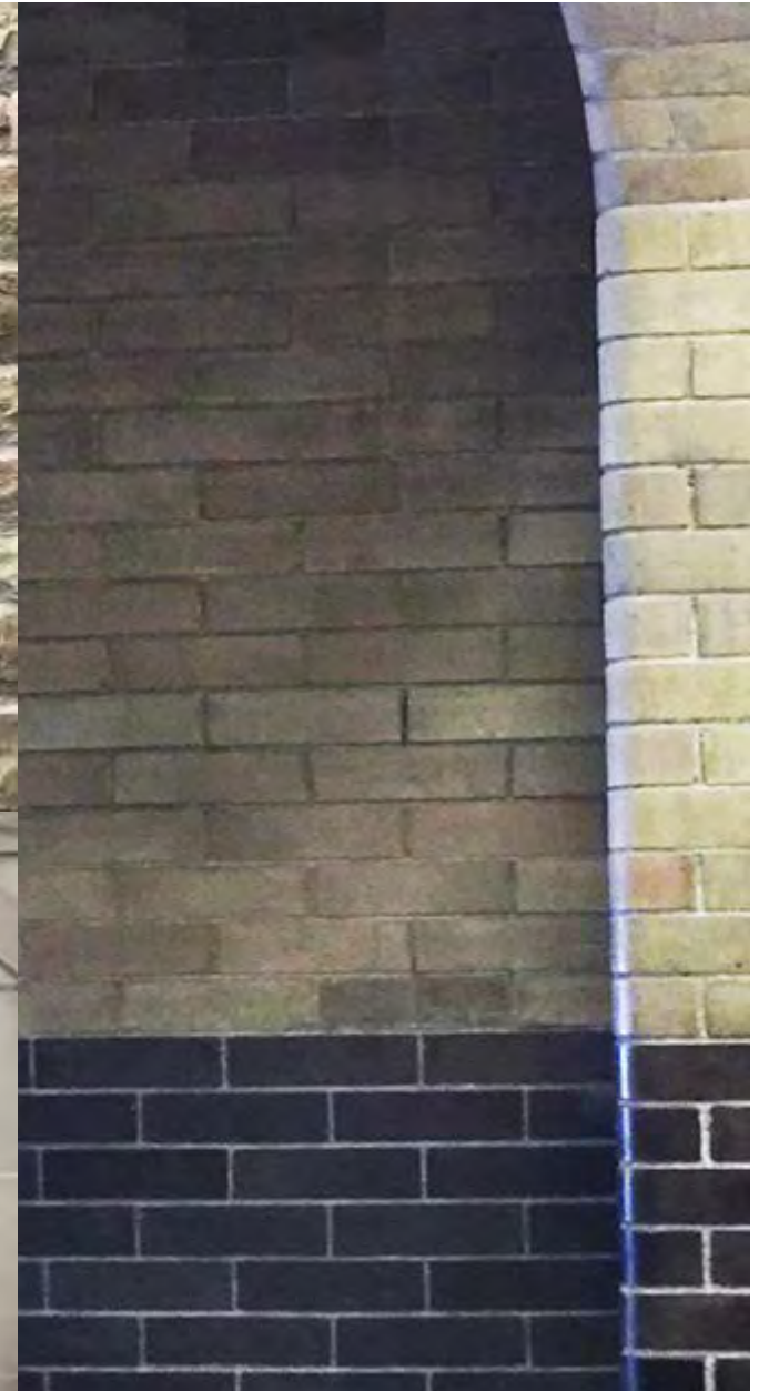
MASONRY WITHIN SCHOOL
