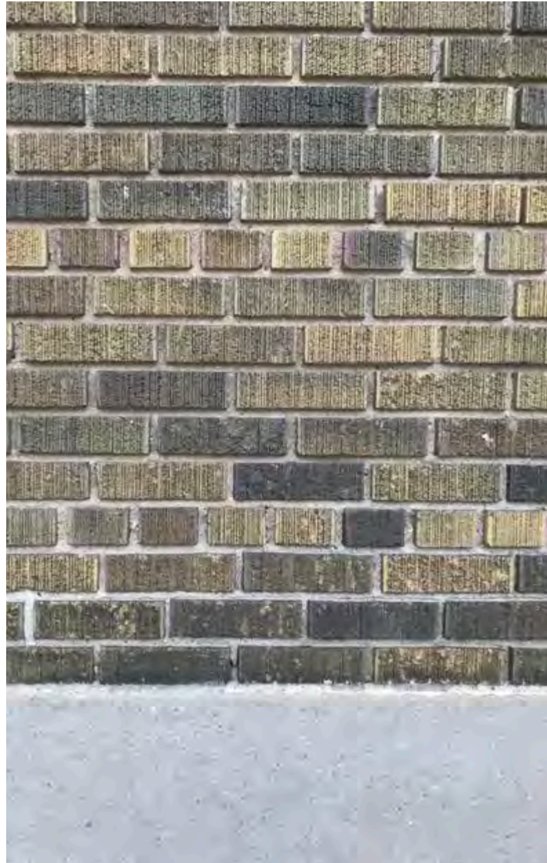
MASONRY AT EXIST. SCHOOL
