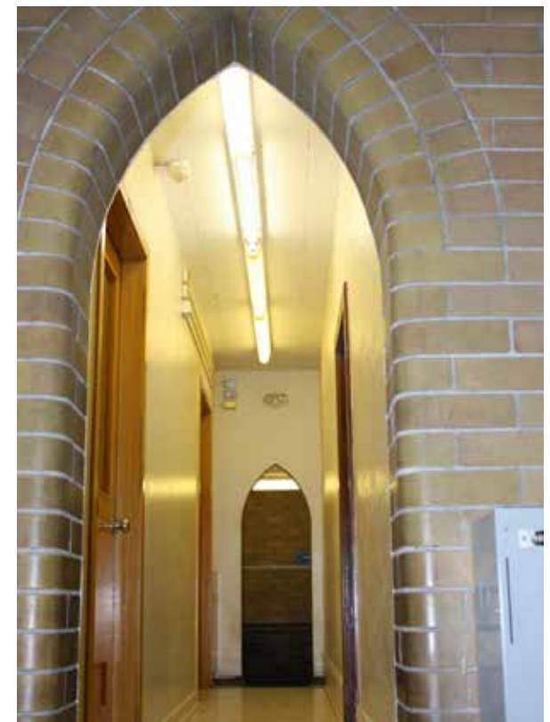
Top to Bottom: Existing 1926 school entry on Stanley Avenue, corridor,
